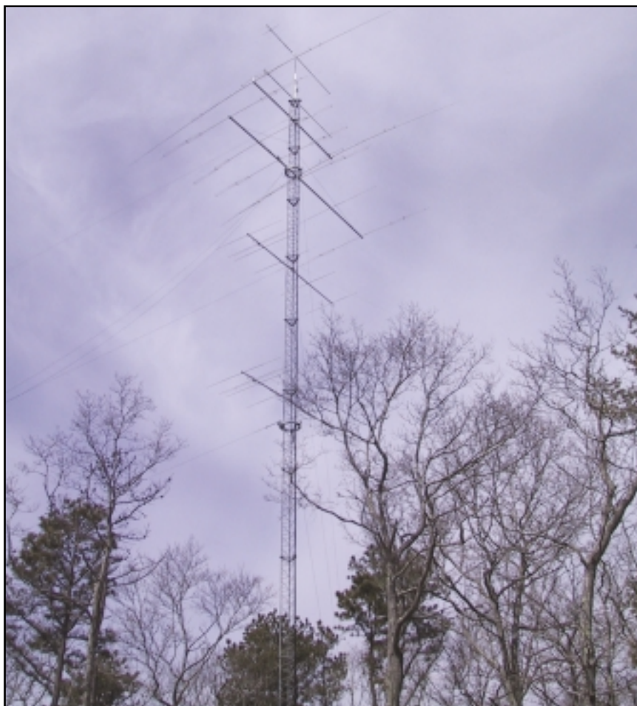
Fig. 1— The author's 100-ft. rotating tower, the subject of this article. Majestic, isn't it? (Photo by KB1LN)
